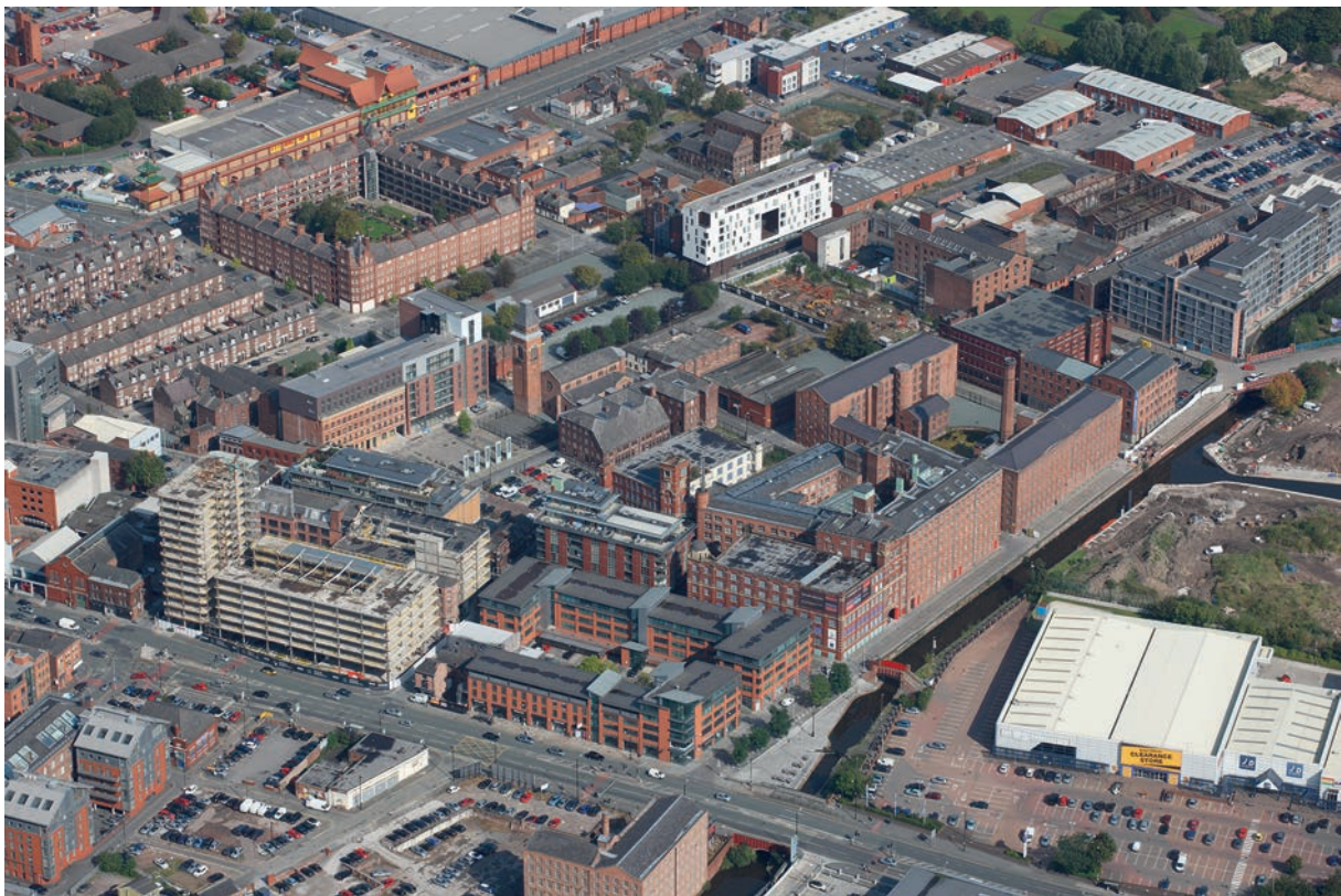
Figure 3b – aerial photograph of Ancoats taken in 2014
